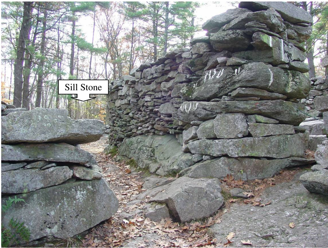
Figure 17 – Current photograph of the Tall Wall’s east side. (Photograph by James Gage)
