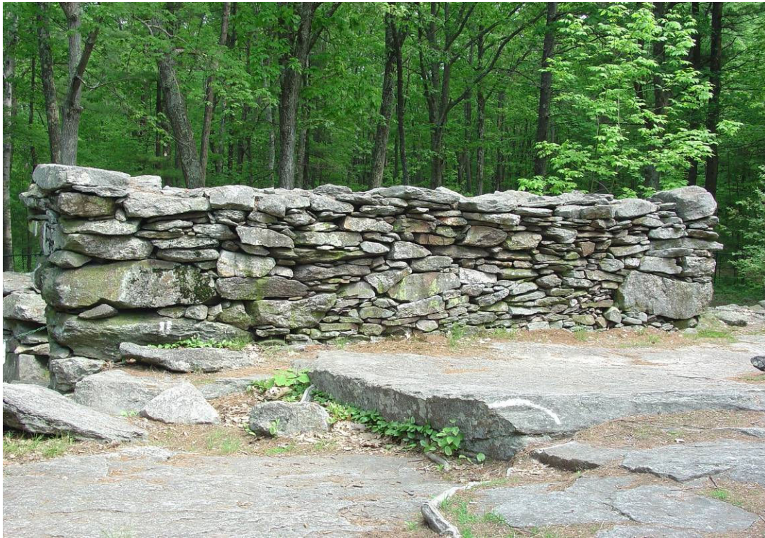
Figure 18 – Current photograph of the Tall Wall’s west side. (Photograph by James Gage)
