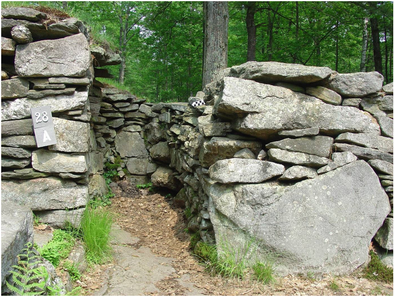
Figure 28 – Current photo of the entrance (alcove) of the Oracle Chamber. The roof stones are missing. (Photograph by James Gage)
