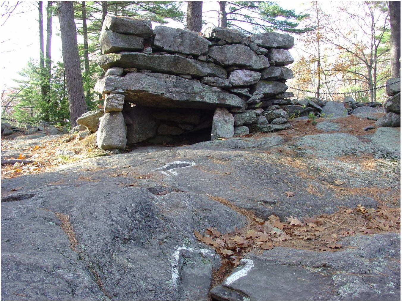
Figure 22 – Current photo of Unnamed Chamber. The section above the roof slab was restored. (Photograph by James Gage)
