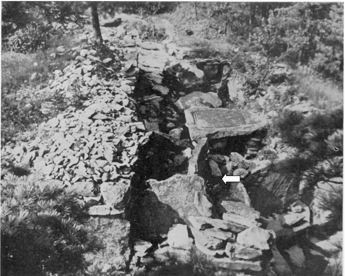
Figure 7 – Photo during restoration. Stones on the bedrock around the Grooved Stone have been placed on top of the Ramp. The upper structure of the Sundeck Chamber is shown (indicated by arrow). (Photo by Malcolm Pearson from Goodwin 1946, 92)
