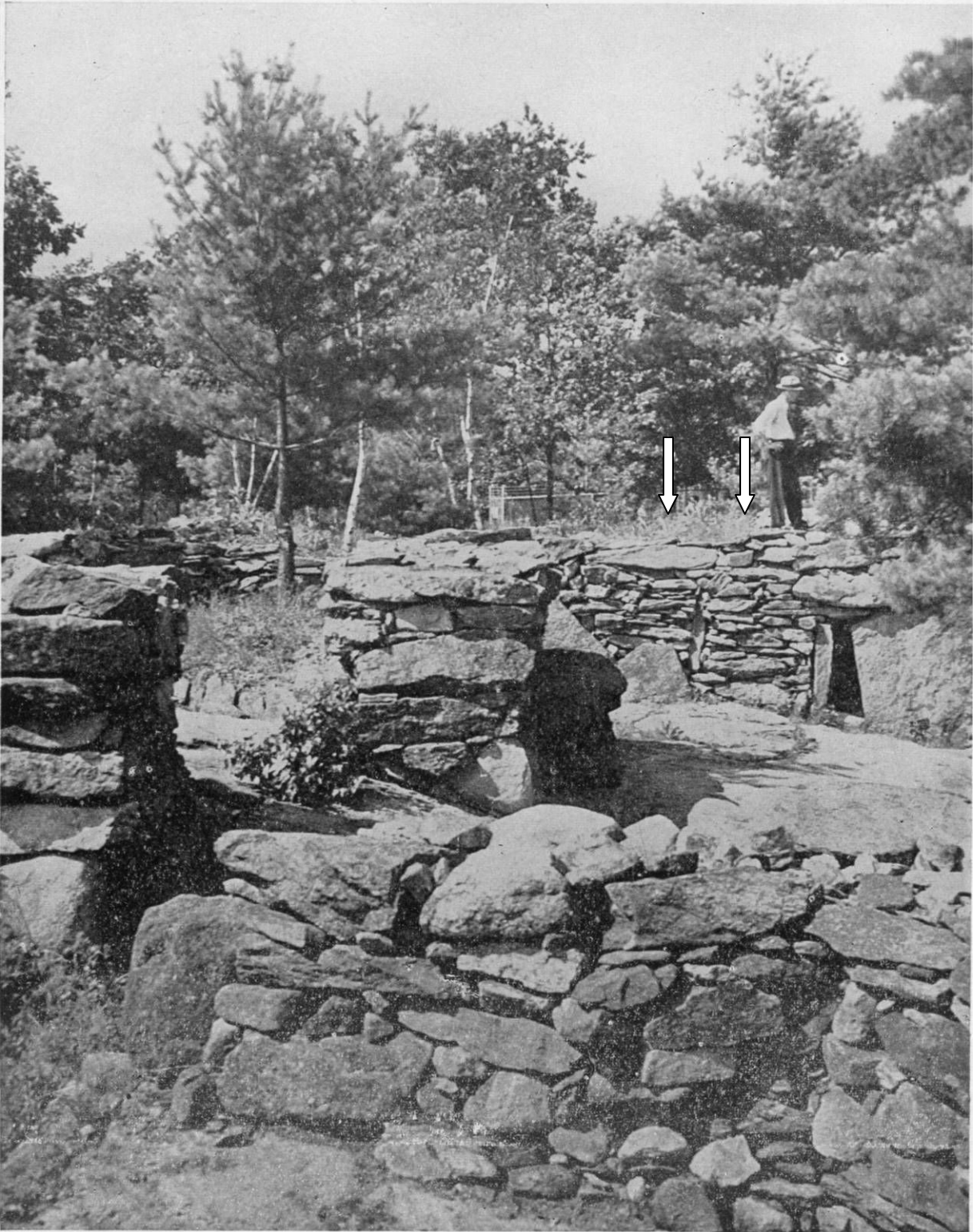
Figure 12 – Post-restoration photo of East-West Chamber circa early 1940s. Middle section rebuilt by Goodwin’s crew. (Photo by Malcolm Pearson from Goodwin 1946, 80)
