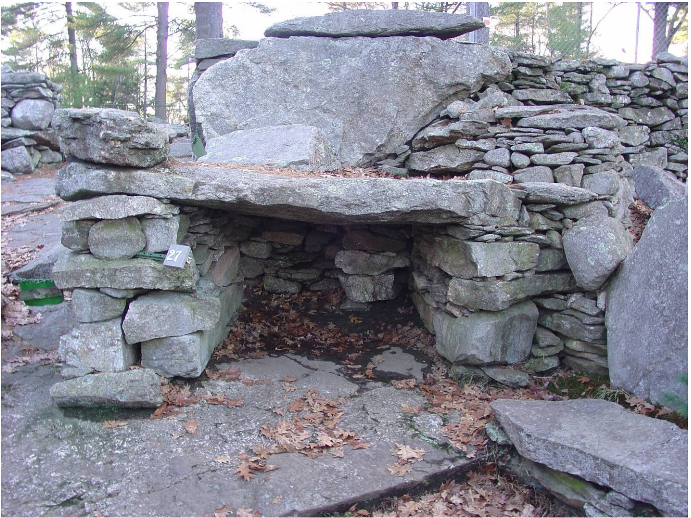
Figure 9 – Sundeck Chamber as it looks today. The left hand support wall has been altered and completely rebuilt. The stones on the upper structure have been re-arranged and does not reflect its original configuration. (Photograph by James Gage)
